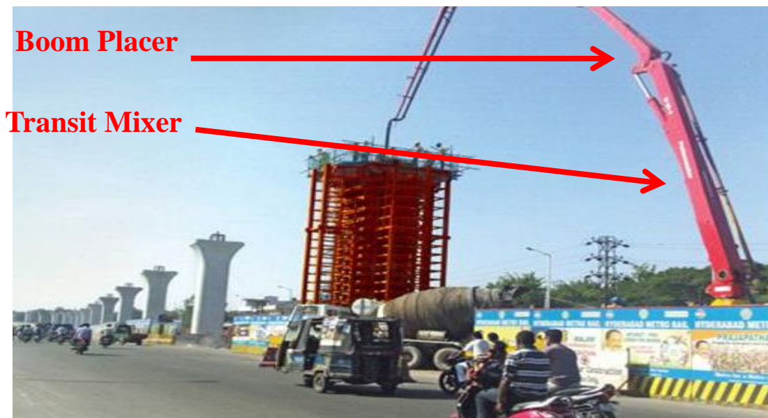
Pier Construction using Boom Placer for evenly filling the concrete
