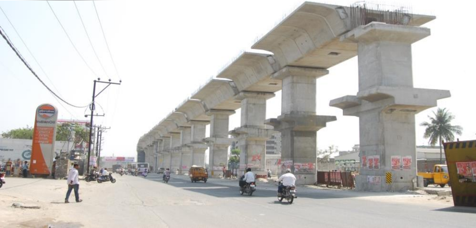
Metro Station Construction-Pier & Segment Stage
