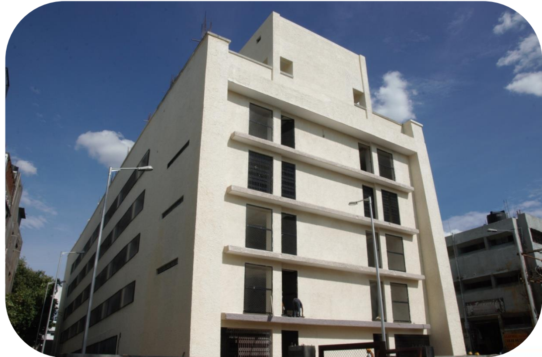
CONSTRUCTION OF PUTLIBOWLI COMPLEX
