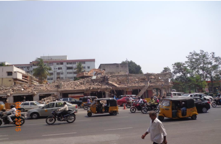
Demolition of Jabbar building
