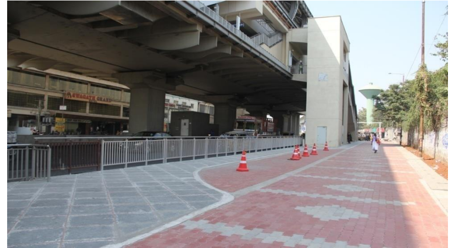
Streetscaping, Parking & Pedestrian facilities, etc., at Habsiguda Metro station
