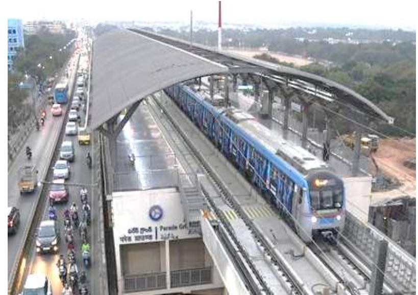
Hyderabad Metro Rail - Typical station
