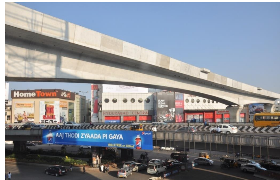
Metro Viaduct crossing flyover
