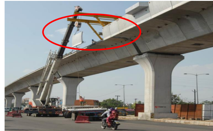
Erecting Parapet Wall on the Viaduct
