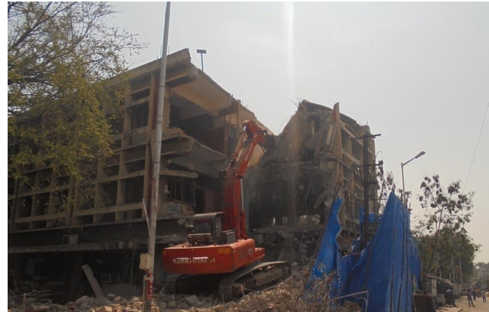
Demolition of BHEL building
