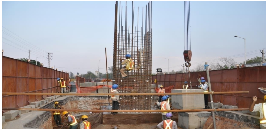
Pier Construction Stage
