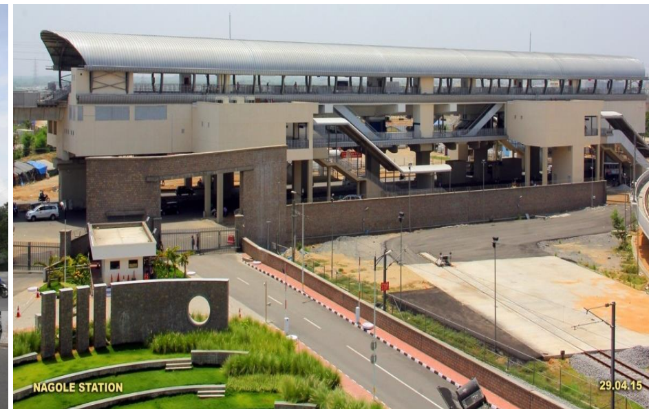
Metro Rail station-Lateral View
