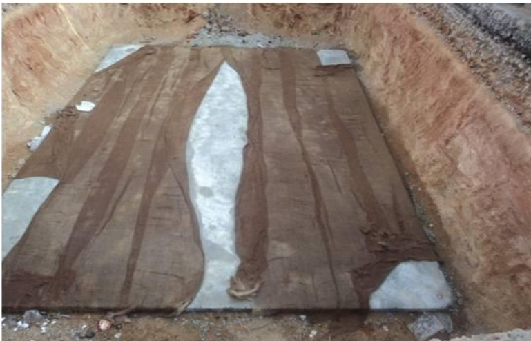
Laying PCC Bed for Foundation – CLSM (Controlled Low Strength Material)
