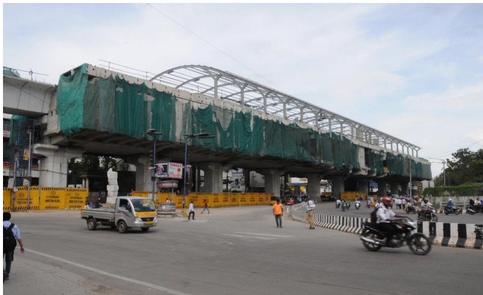
Metro Station Construction-Roofing Stage
