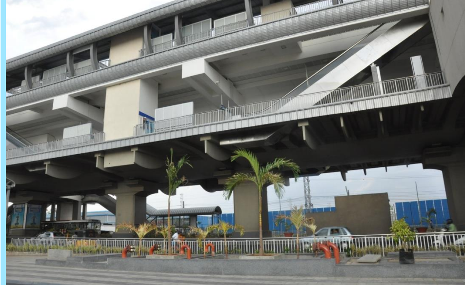
Cantilever type Metro station resting on the central pillars
