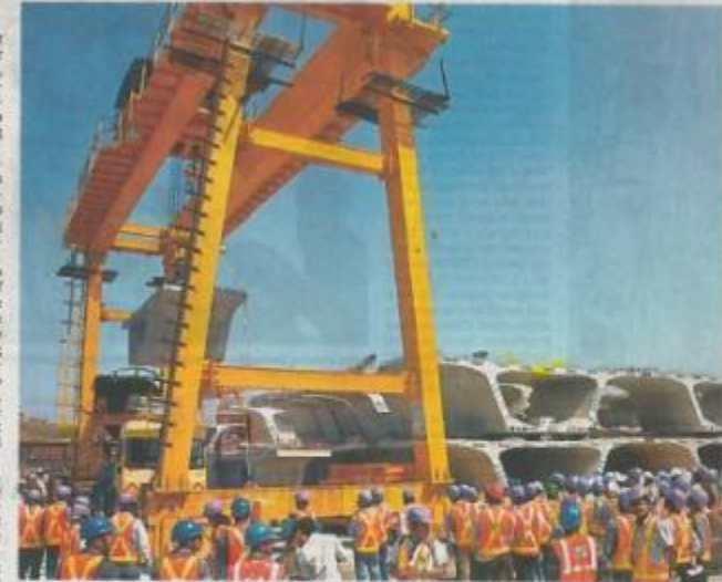
Viaduct segments for Hyderabad Metro Rail project being manufactured at Quthbullapur casting yard in Hyderabad on Tuesday | enr.in
