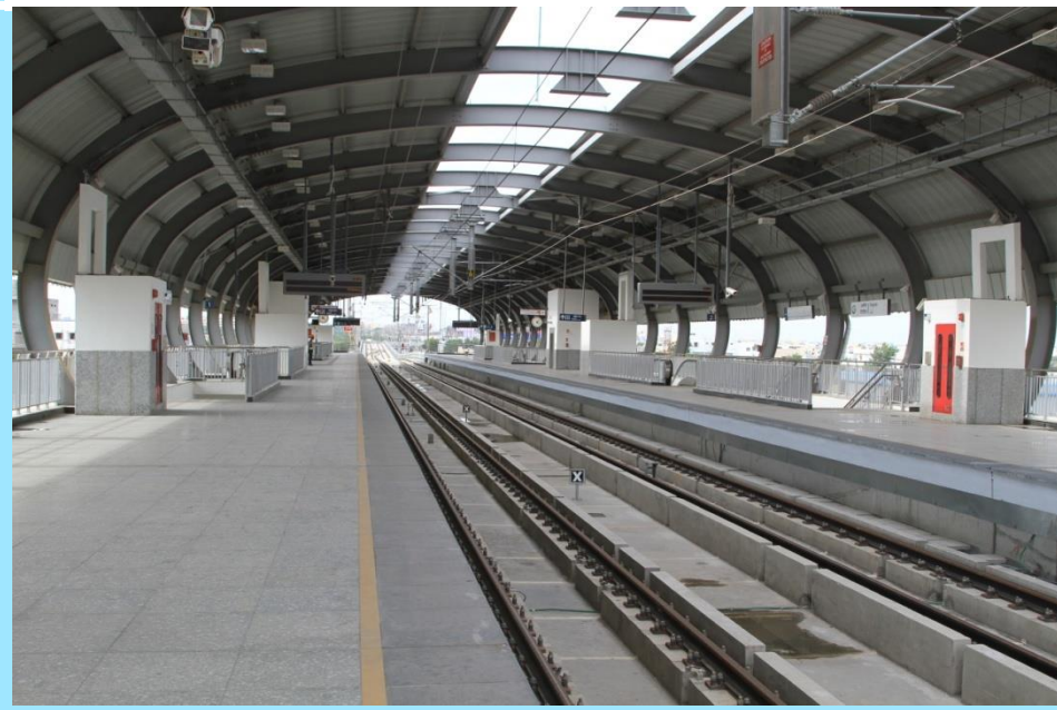
Platform level of Metro Station
