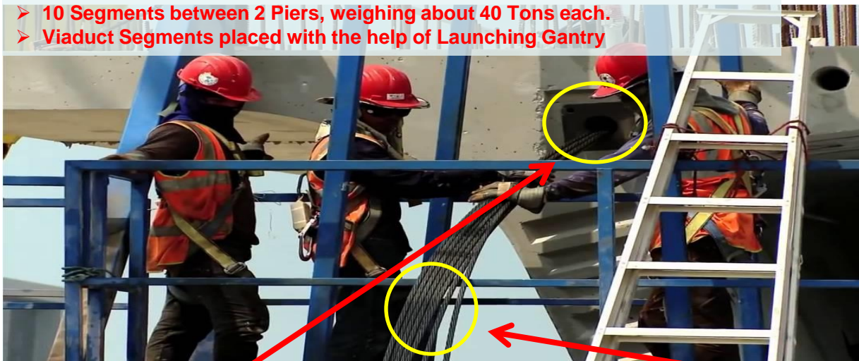
Duct in Pre-Cast Segment
