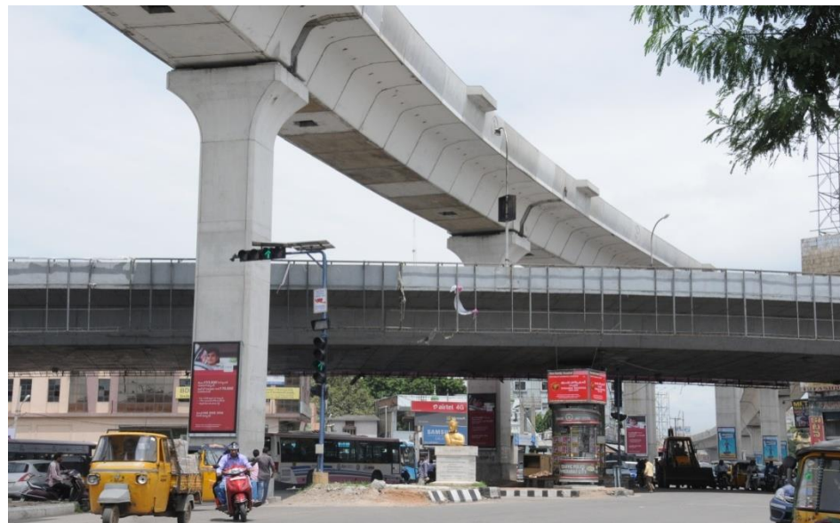
Metro viaduct crossing at Malakpet flyover
