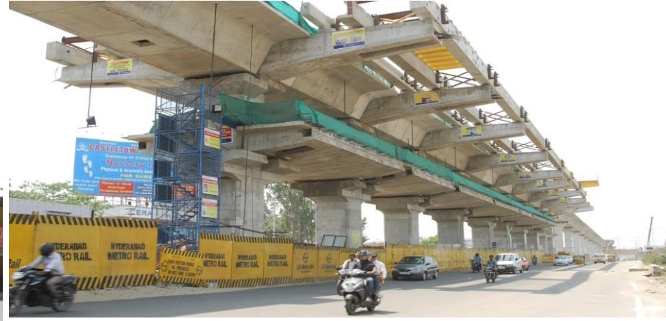
Metro Station Construction-Spine & Wings Stage
